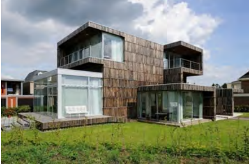
Fig. 12 - Welpeloo House in Enschede, The Netherlands.
