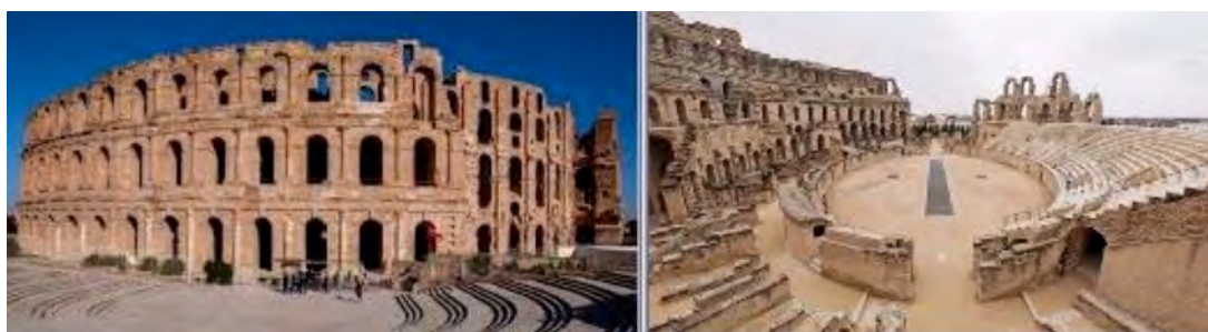
Fig. 4 - El Djem Arena. An external view (left) and an internal view (right).
