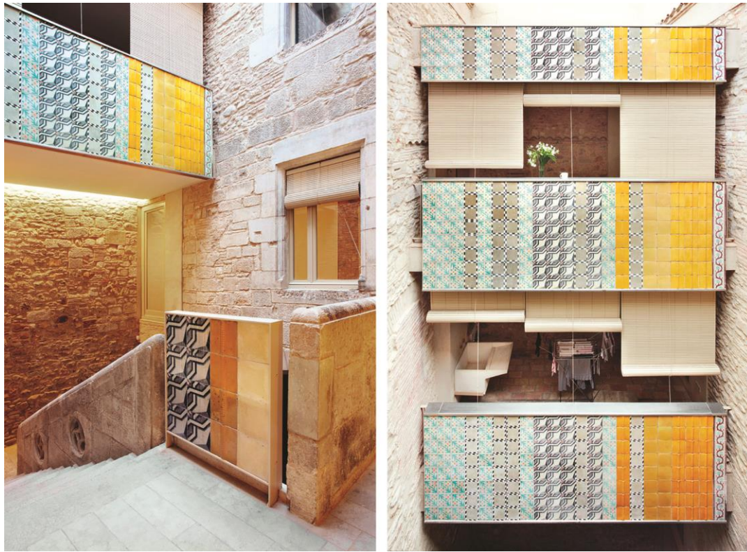
Fig. 9 - Bosch.Capdeferro architecture, Casa collage. Reuse of reclaimed ceramic pieces, mosaics and stones in a refurbishment: views of the inner patio. Girona, Spain, 2009. Credits: José Hevia.
