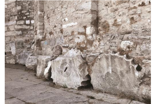
Fig. 3 – Pedestals of ancient columns included in the external walls with indifference towards their previous function, Church of St Donatus, Zadar. Credits: the authors.
