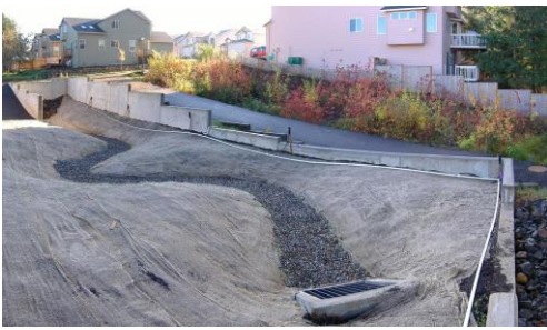
Fig. 3 - An example of SUDS under construction (foreground) and established (background) (Source: @Duk at English Wikipedia)
