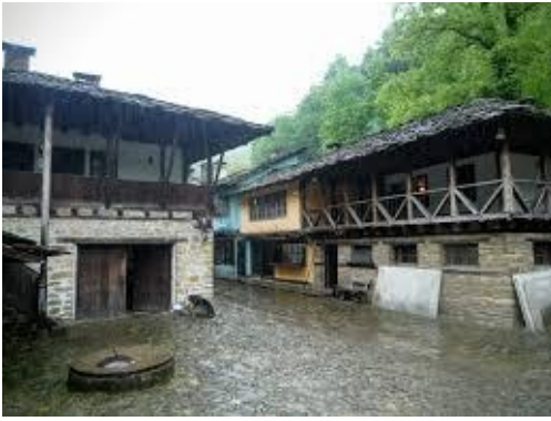
Fig. 2 - Architectural Ethnographic Complex Etera, near town of Garbovo, Bulgaria
