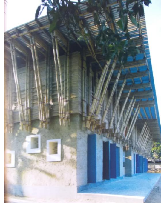
Fig. 4 - Rammed earth walls
