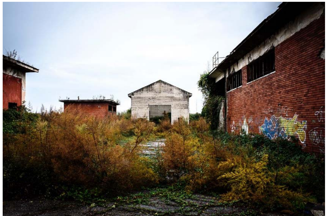
Fig. 1. Abandoned peri-urban areas in the Metropolitan Area of Naples (photo credits: Alessandro Capozzoli).
