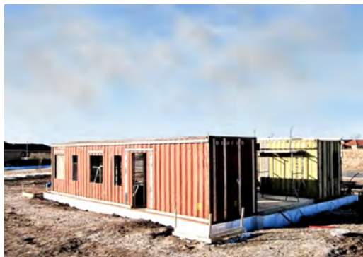
Fig. 16 - Upcycle House, Lendager Arkitekter - Nyborg, Denmark, 2013. Containers used for the structure
