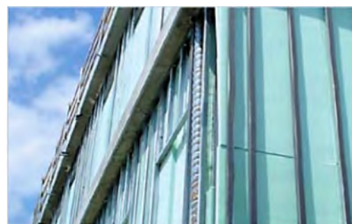
Fig. 9 - Savno' s building, Conegliano, 2008. Thermal and acoustic insulation panels made of recycled PET. Available at: www.savnoservizi.it
