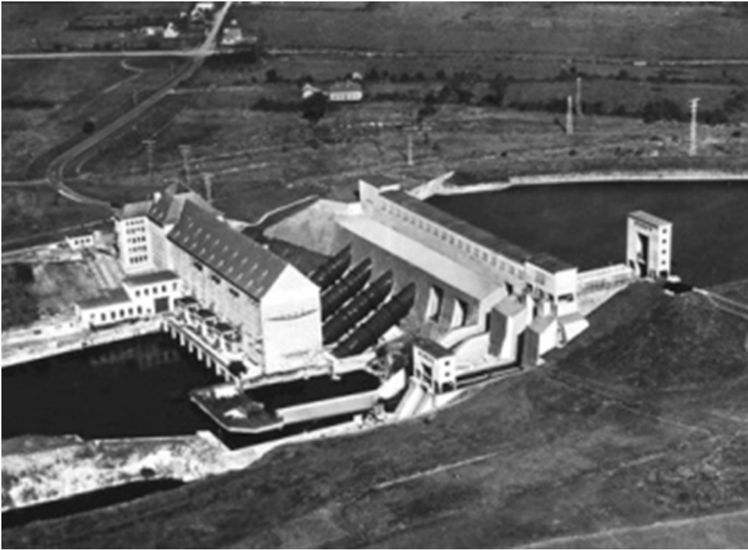
Fig. 3 - General view of the Ardnacrusha hydroelectric power plant on the Shannon, 1929.
