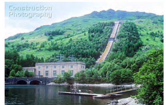
Fig. 12 - A hydro electric power station on the shores of loch Lomond, Scotland, UK.
