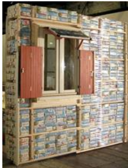
Fig. 6 - STONE module in Legnano. The walls with Tetra Pak cases. Photo by A. Rogora
