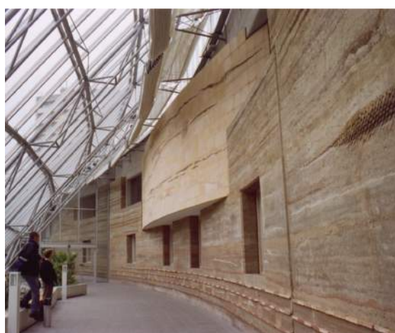
Feldkuch Regional Hospital, designed by G.Grass; arch.E. Gutmorgeth; arch. A.Kuthan; arch M.Rauch (M.L. Miccoli)
