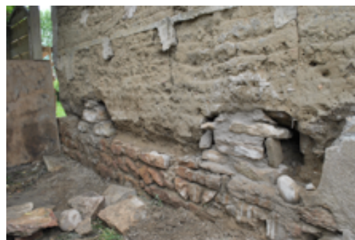
Fig. 2 - Raising the stone basement.
