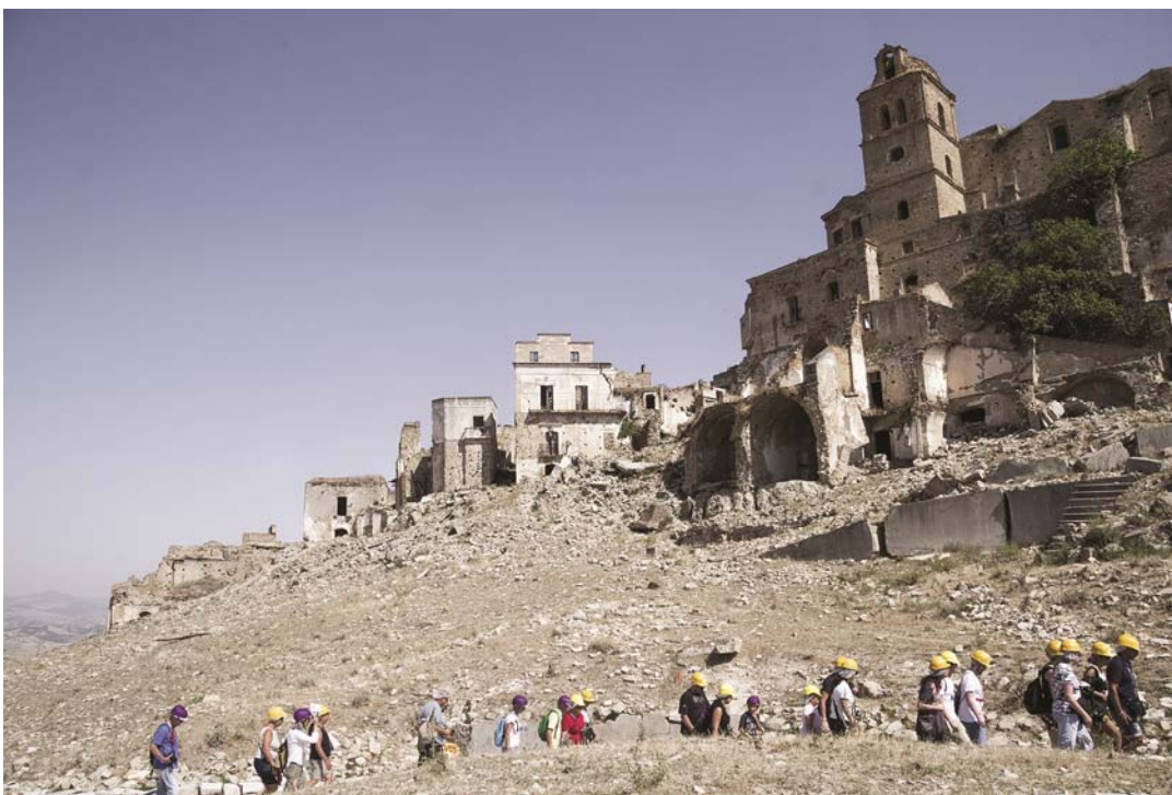
Fig 3. The ghost village of Craco. Guided tour in safety in august 2019 (photo credits: P. Zizzania).
